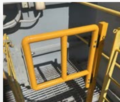
Controlled access, preventing unauthorised entry, and enhancing employee safety
