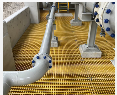
Precise offsite fabrication, quickly installed, minimising downtime and enhancing operational safety
