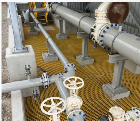
FRP pedestal-supported grating provides a safe, and elevated walkway
